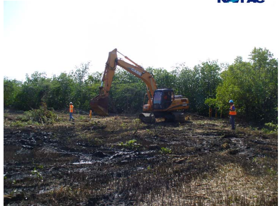
Waste removal (10 Feb 09)
