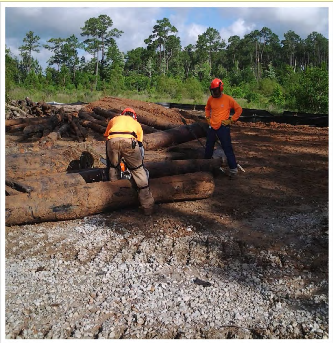
Timbers from the haul road being cut and readied for transport off site.
