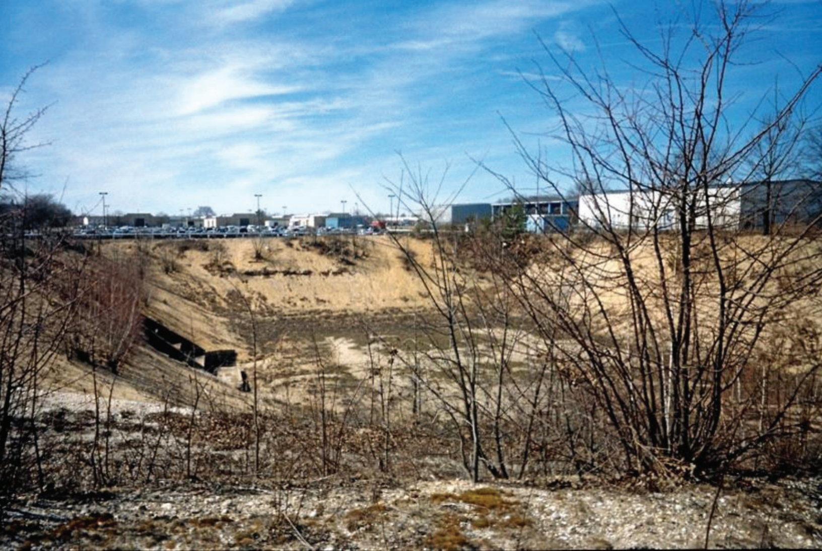
(Above) Recharge Basins at Site 2 which used to temporarily store runoff. Recharge Basins release at least a portion of runoff by infiltrating water into the ground. The recharge volume is stored and allowed to infiltrate into the underlying soils over a period of time following a storm event (see below example). The storage volume above this level may be released by an outlet structure designed to bypass all excess flows.
