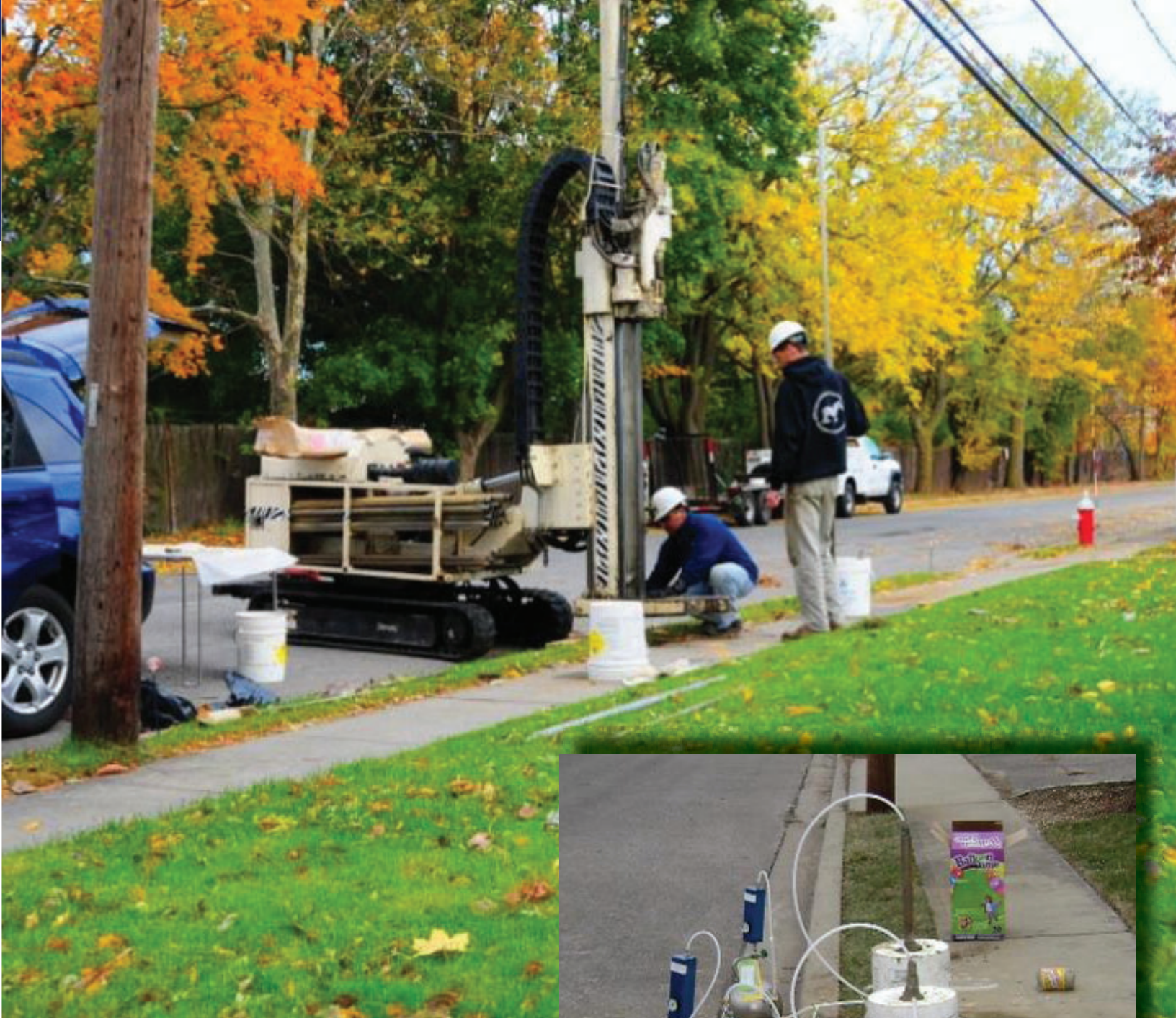
(Above) Technicians perform Soil Gas Sampling in a Nassau County residential neighborhood. Soil gas can be tested in different ways. The most common method uses a hollow metal rod that is inserted into the soil. To measure the soil gas holes are drilled and the rod is pushed into the soil. A pump draws the soil gas through the hollow rod into a sampling container or canister. The gas is then either analyzed by the testing equipment on-site or the sampling container is brought to an off-site laboratory for analysis.
