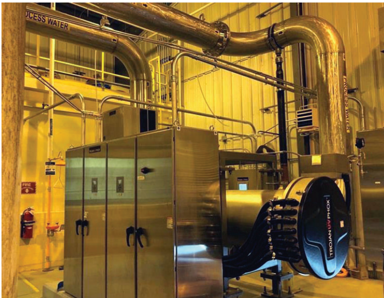
(Below, right) A technician operates the Operable Unit 2's, Advanced Oxidation Process Reactor (left) for 1,4-Dioxane Treatment, GM38 Area Hotspot Treatment System for the Recharge Basin (above).
