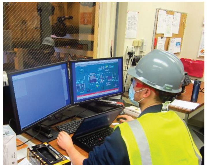
(Below, right) A technician operates the Operable Unit 2's, Advanced Oxidation Process Reactor (left) for 1,4-Dioxane Treatment, GM38 Area Hotspot Treatment System for the Recharge Basin (above).
