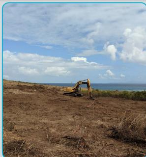
**Using a remote-controlled excavator to rake vegetation in the Submunitions Area**
