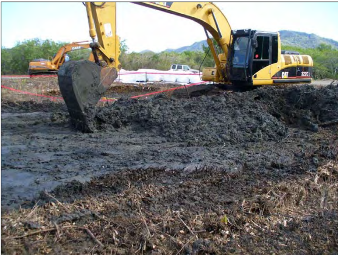
Scraping of debris and soil from the surface of SWMU 6 (2/13/2009)
