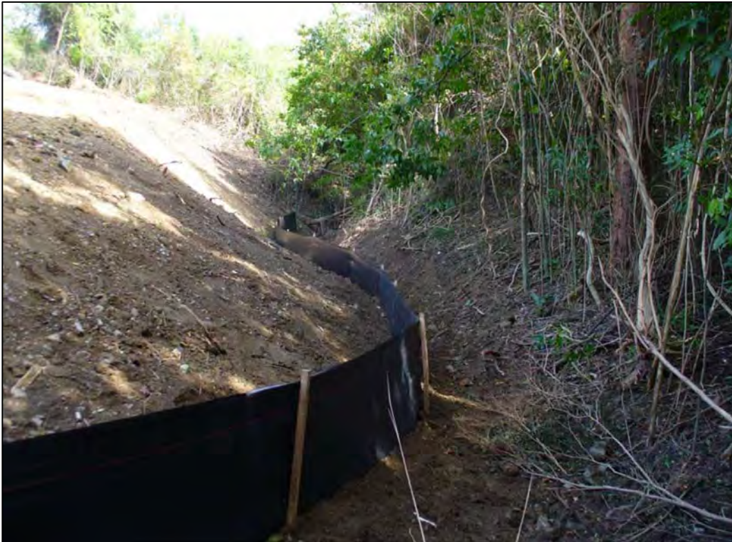
Looking along the base of slope at the silt fence installed following the removal of all debris at SWMU 7 as of February 2009. (2/20/2009)
