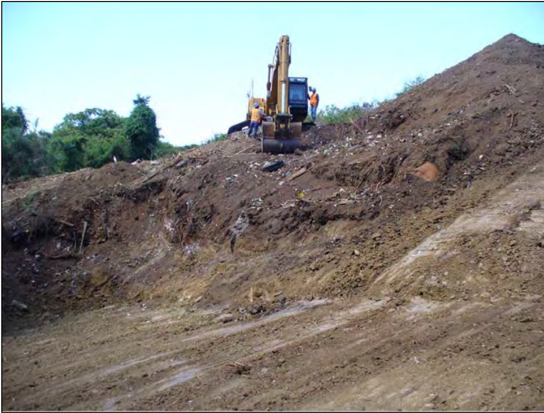
Looking up the slope as debris is removed at SWMU 7. The area in the foreground has been scraped clean of debris. Image shows site conditions during remediation. (2/13/2009)
