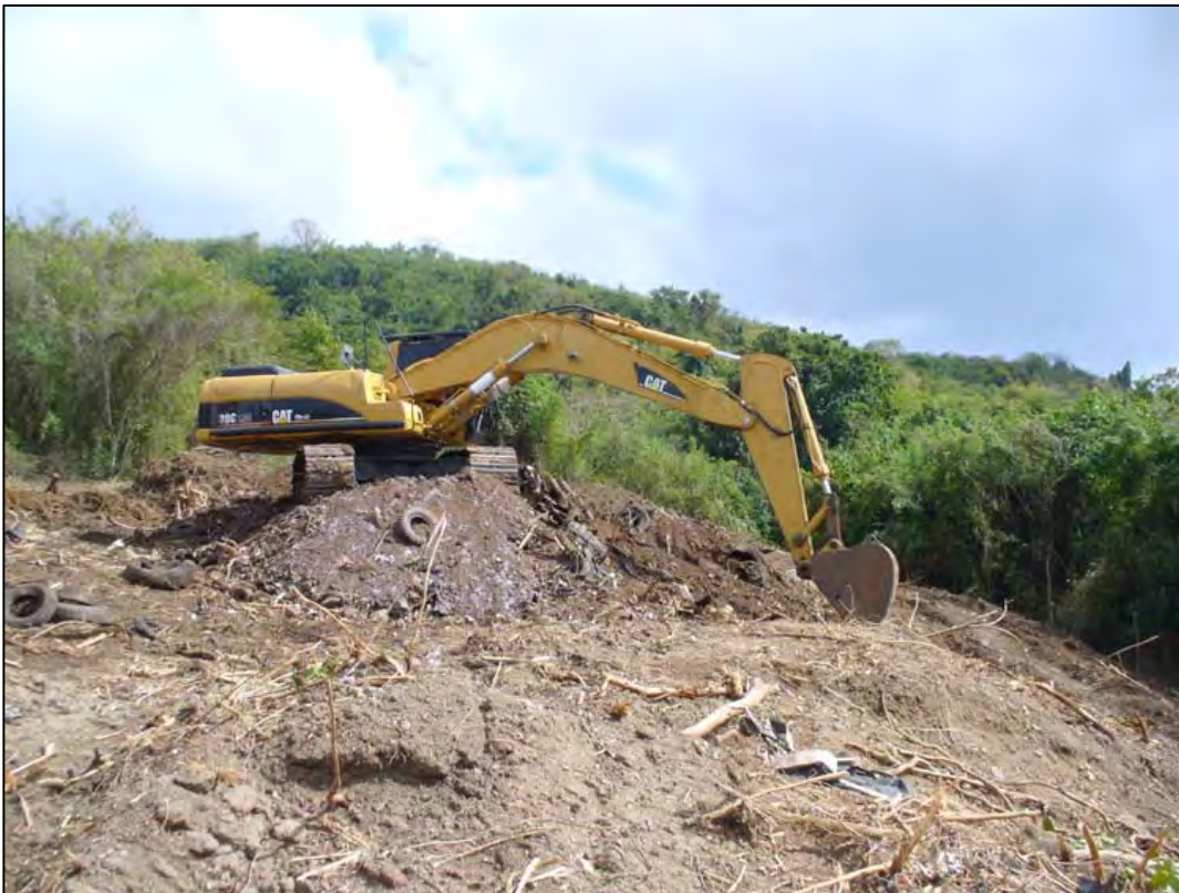
An excavator consolidating small sized debris and soil for transport to the staging area at SWMU 7. Image shows site conditions during remediation. (2/11/2009)
