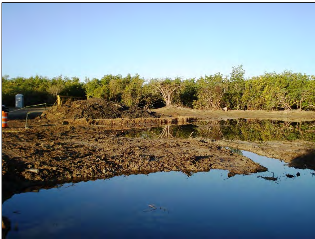
Looking toward the west at the site following excavation. Excavated soil is staged on plastic sheeting and surrounded by hay bales. (4/3/2009)
