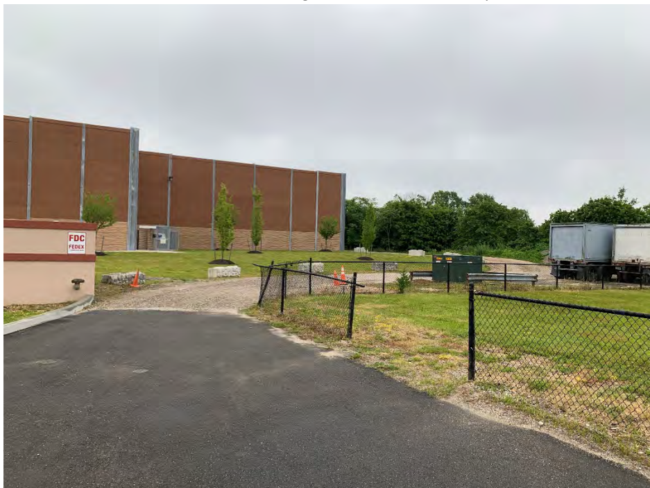
Photo 2B – Southwest corner of Site 2 looking northeast at FEDEX facility sound walls
