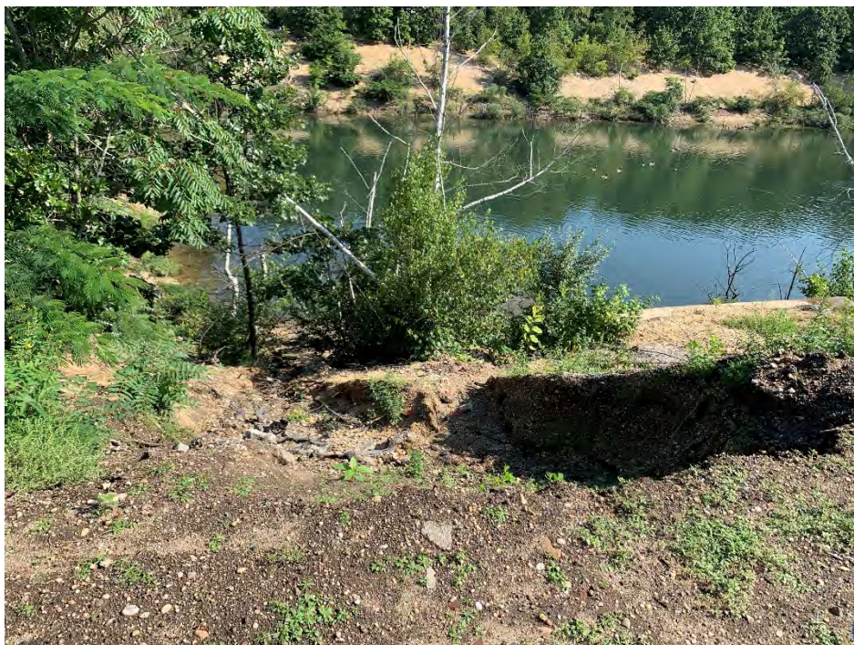
View looking north at area of erosion on the northeast recharge basin
