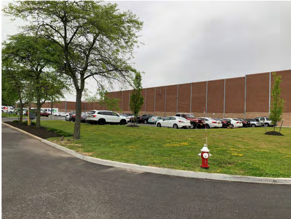
Photo 3C – Southeast corner of Site 3 facing northwest showing the FEDEX hub terminal sound walls and southern parking area
