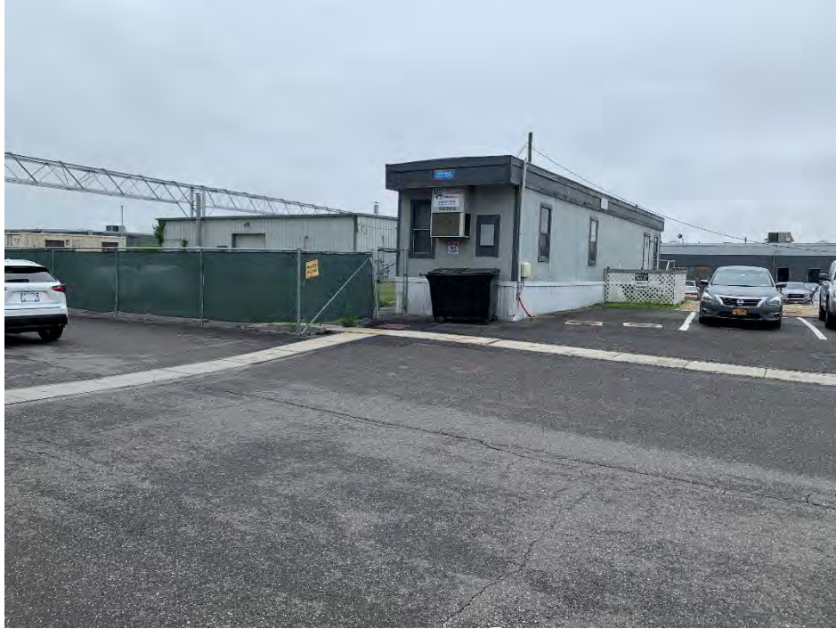
Photo 4B – Northwest corner of Site 4 facing southeast looking at Navy trailer, warehouse and fenced in area
