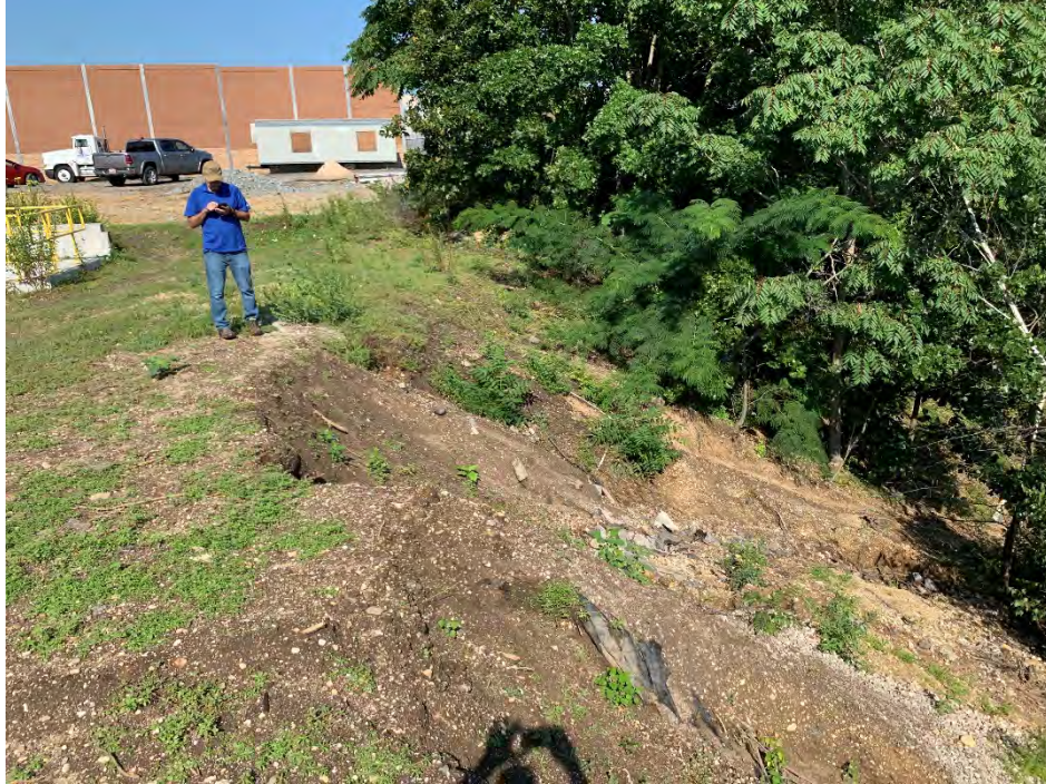
View looking west at area of erosion
