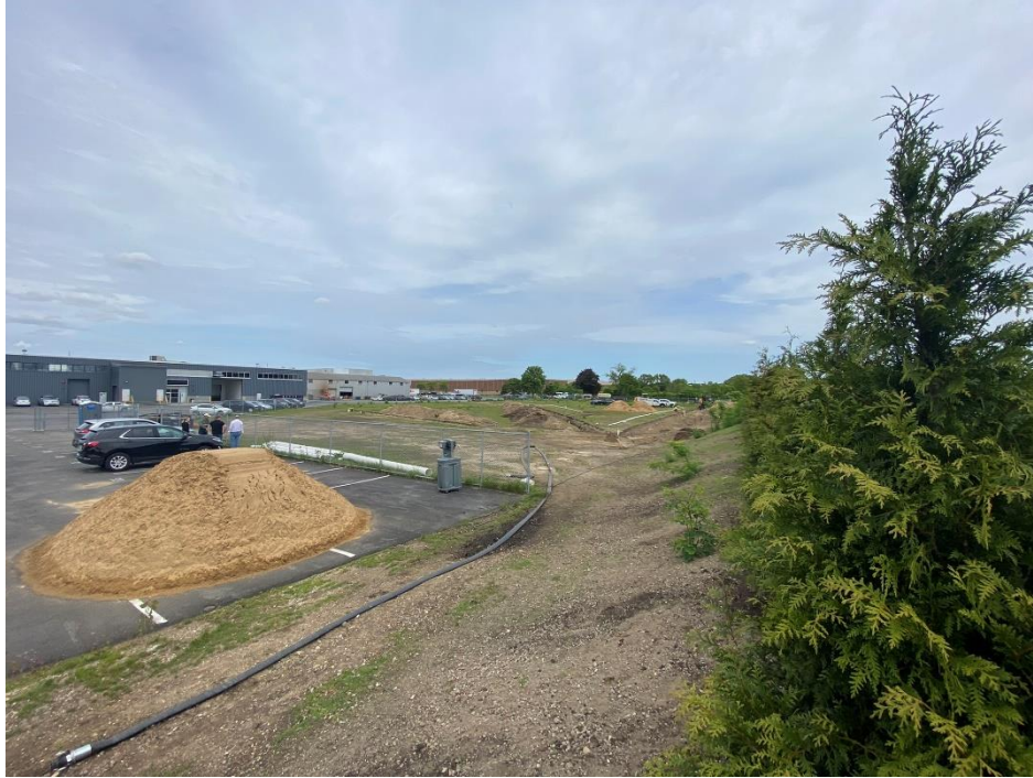
Southwest corner of Site 1 looking northeast at center of site, trenching in place for new SVE piping
