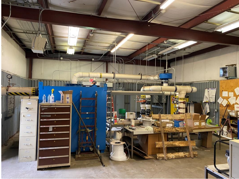
View of Site 1 SVE system blowers and GAC unit
