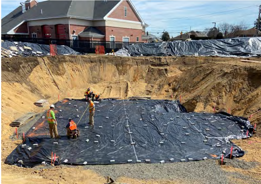
March 15 th , 2022. field crews marking out the locations for footing forms within the sump area in northern portion of water treatment plant footer. Looking east.
