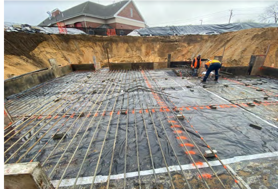
March 18 th , 2022. Initial stages of rebar installation within the sump area in northern portion of water treatment plant footer. Looking east.
