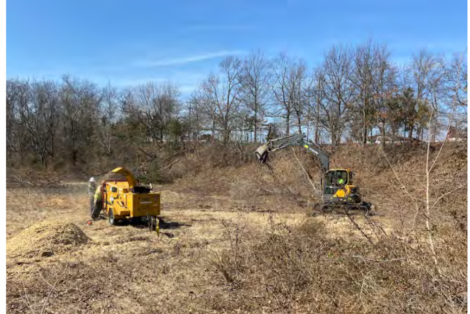
March 14 th , 2022. Initial stages of clearing and grubbing within Nassau County Basin N477. Excavator being used to move cut organic debris to woodchipper. Looking north northwest.
