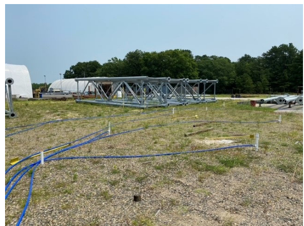
Biosparge System at Site 7
