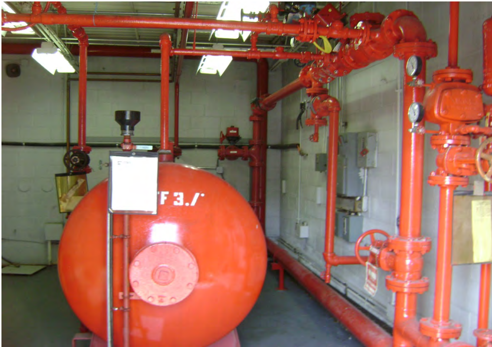
Photo 1 - Building 327 - Tank with FFFP
