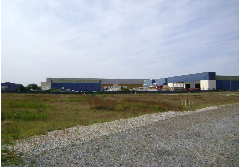
Photo 10 - Buildings 06-15 [168] and 06-66 [318] – Aircraft Paint Hangars and Site 6A – Former Fuel Calibration Area, Looking west
