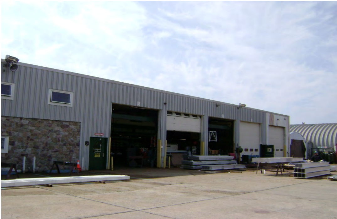
Photo 8 - Building 07-04 (283) – Flight Emergency Shelter (Fire House), Looking South West
