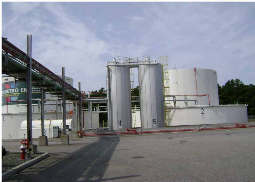
Photo 4 - Looking West of Building 327 – Fire Suppression Piping
