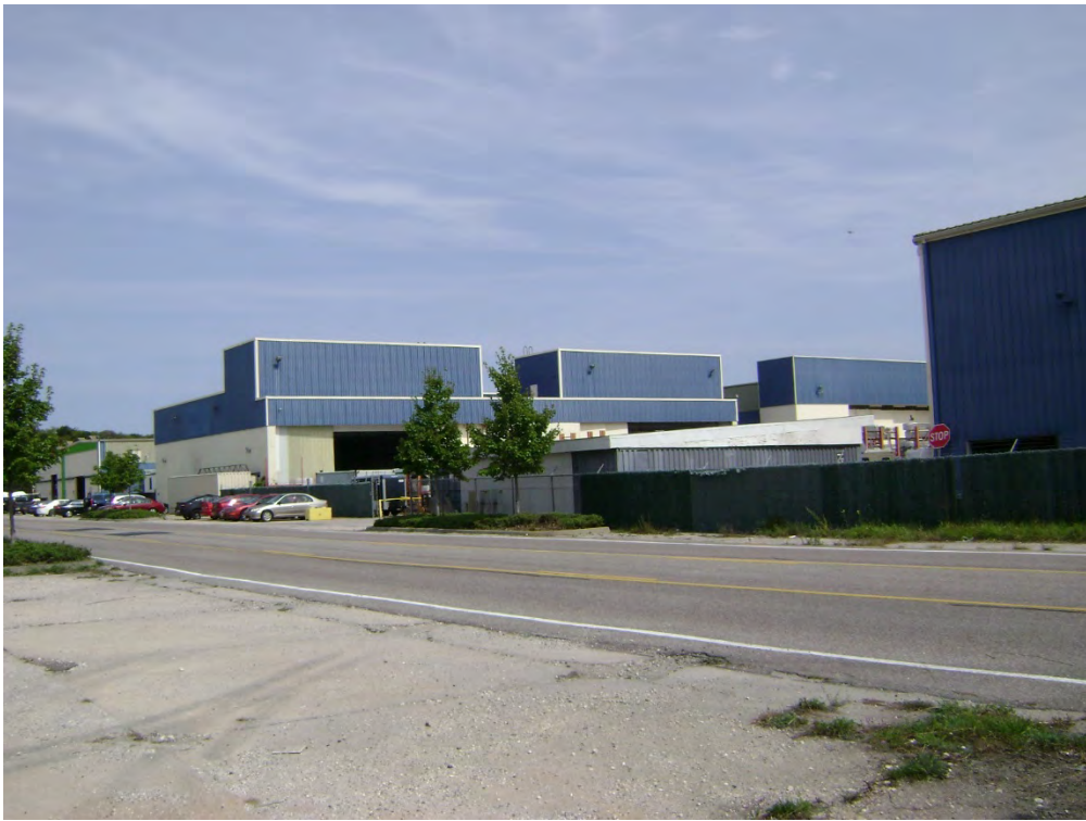
Photo 9 – Buildings 06-15 [168] and 06-66 [318] – Aircraft Paint Hangars, Looking East
