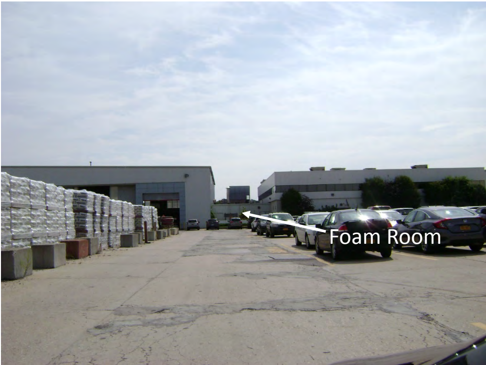
Photo 6 – Buildings 81-5, 6, 7, and 8 – Foam Room, Looking South East
