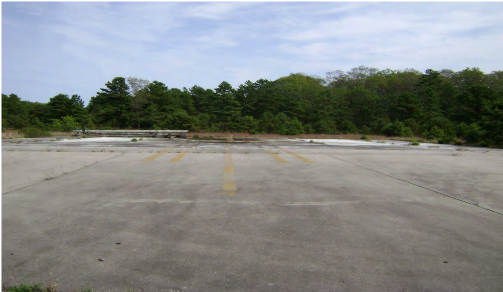
Photo 12 - Building 06-79 – Noise Suppression Hush House, Looking East
