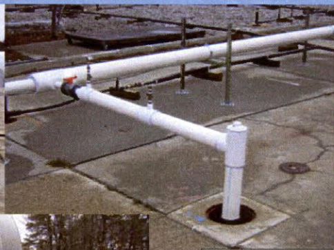
Typical SVE Well Head Connection
