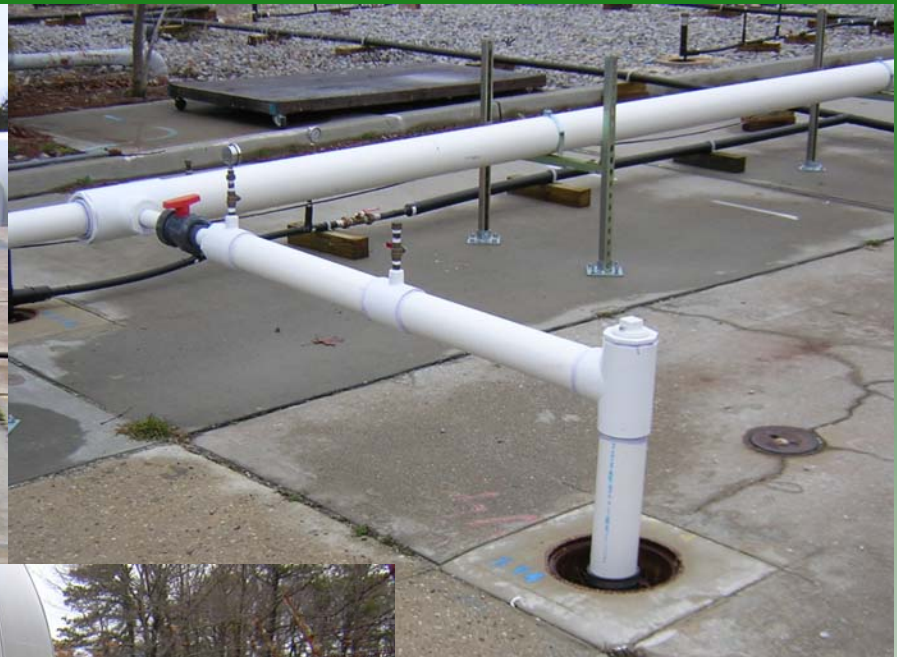
Typical SVE Well Head Connection
