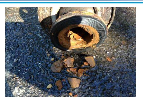
FLTS effluent discharge pipe prior to rehabilitation. Build up of iron precipitate inside discharge line. Effluent line was cleaned, resulting in increase discharge capacity.
