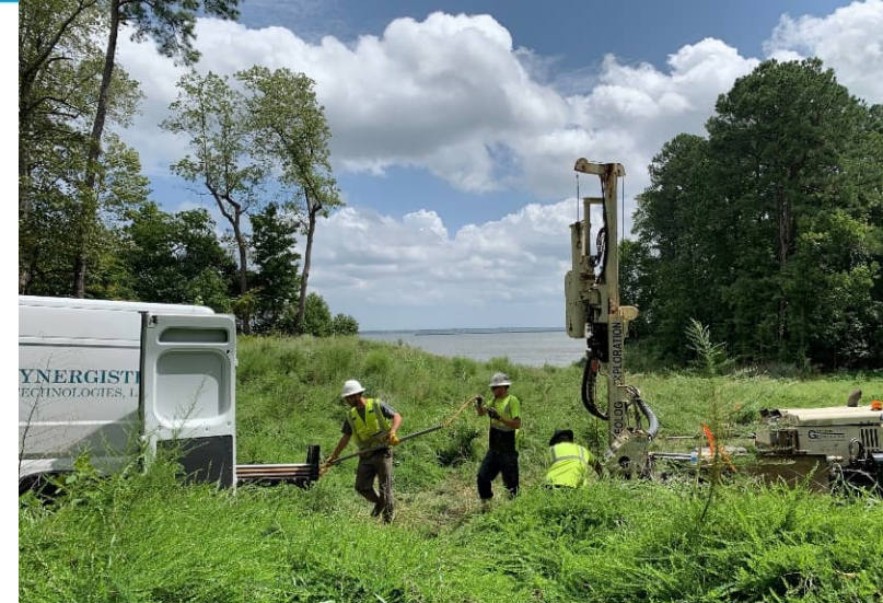
Hydrogeological data collection with HPT tooling
