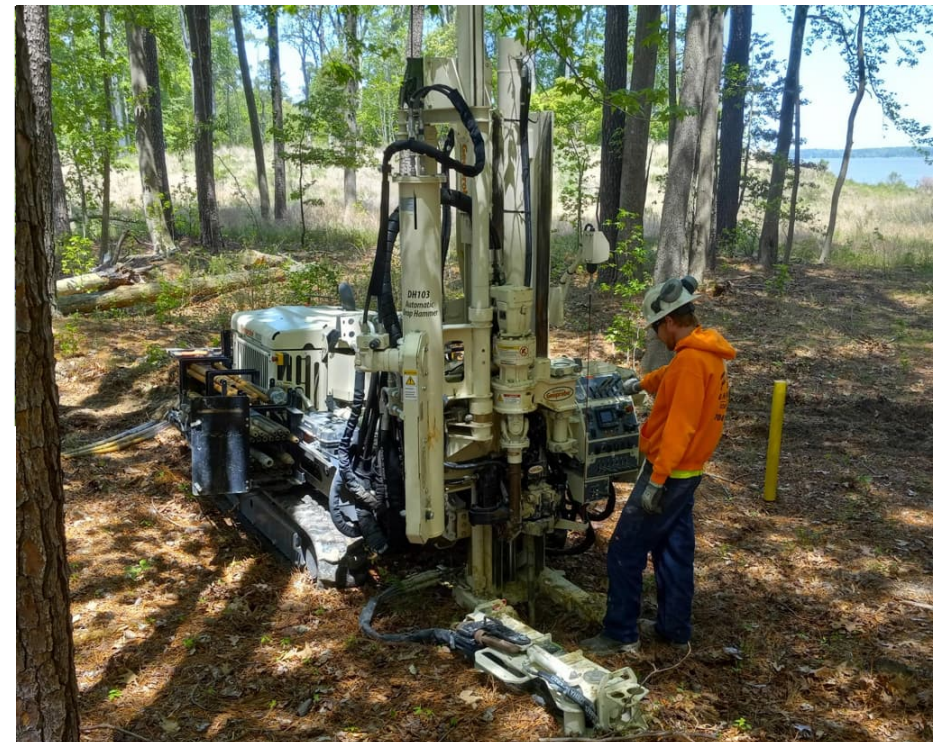
Groundwater sample collection with DPT rig
