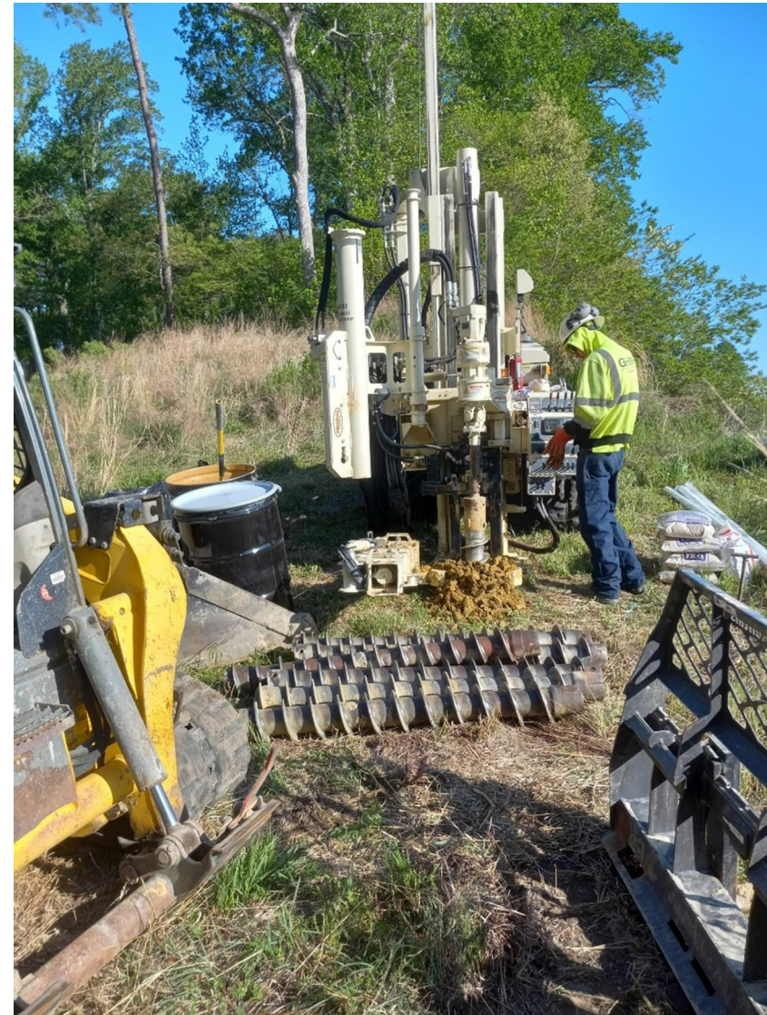
Installation of groundwater monitoring well
