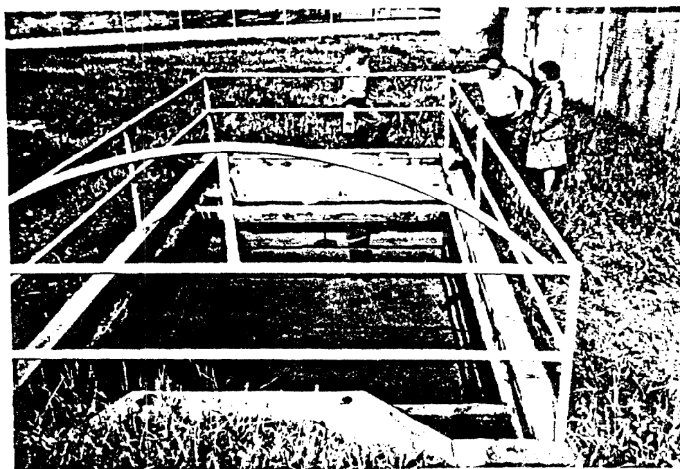
Figure 6.1-2 Sump for Bldg. 126
