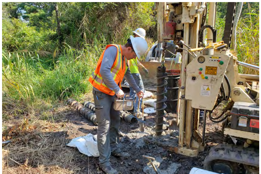
Monitoring well installation at Regulus Avenue Landfill, Dam Neck Annex
