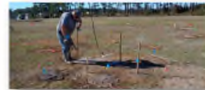
A new treatment technology being used at Site 6 involves injecting materials into the soil and groundwater to help release oxygen. The increased oxygen can help break down hydrocarbons present at the site.
