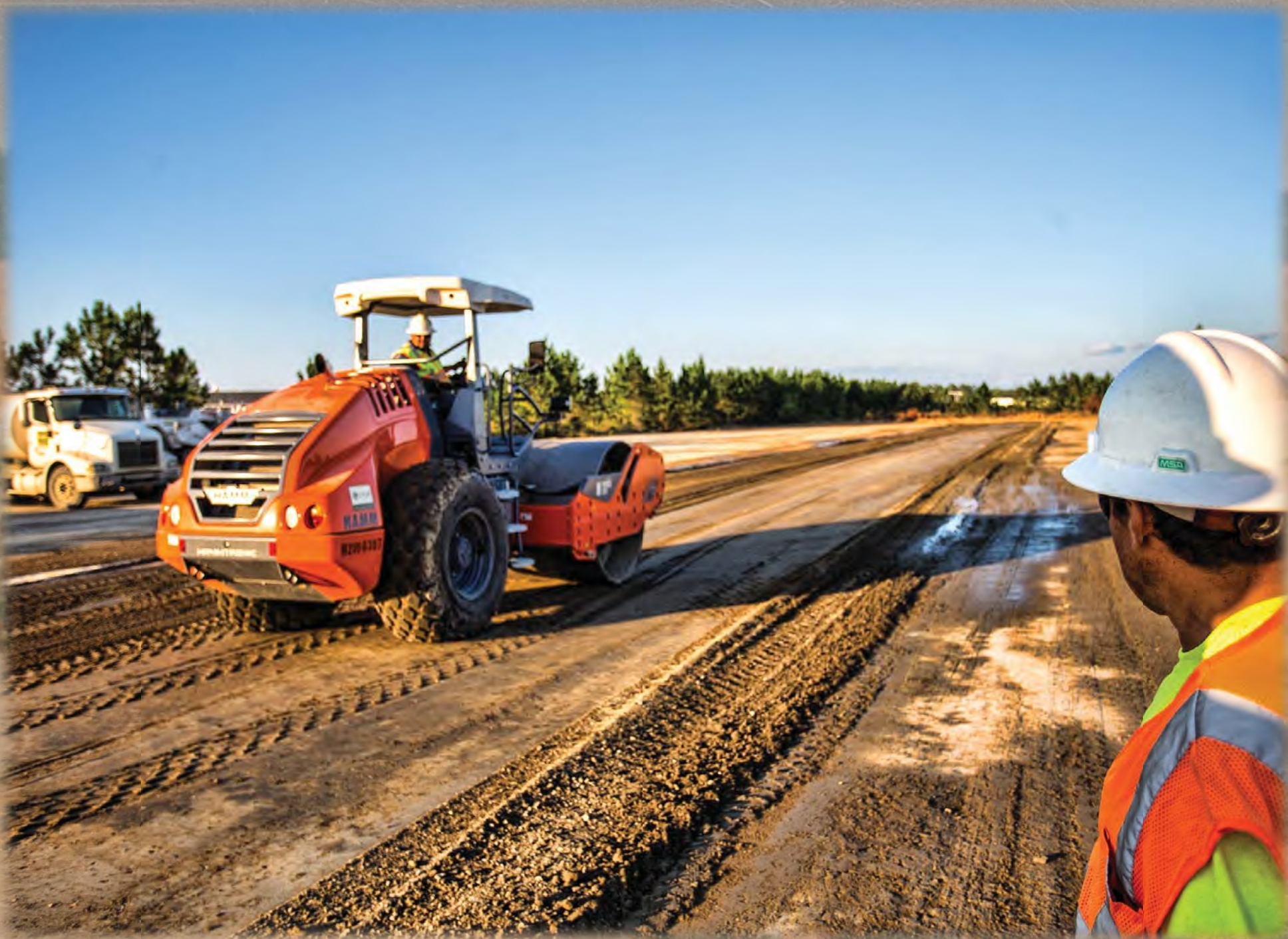
Compacting Milled Cement/Sediment Mixture for Final Stabilization
