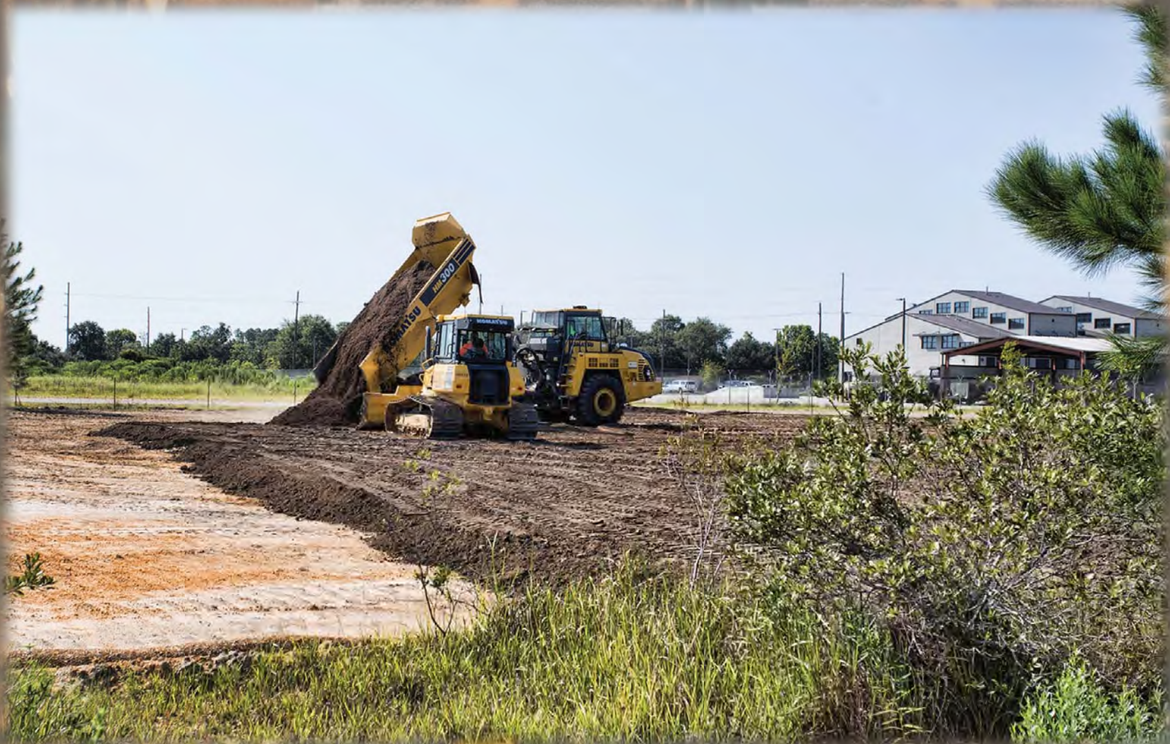
Application of Screened Sediment to Stabilization Area
