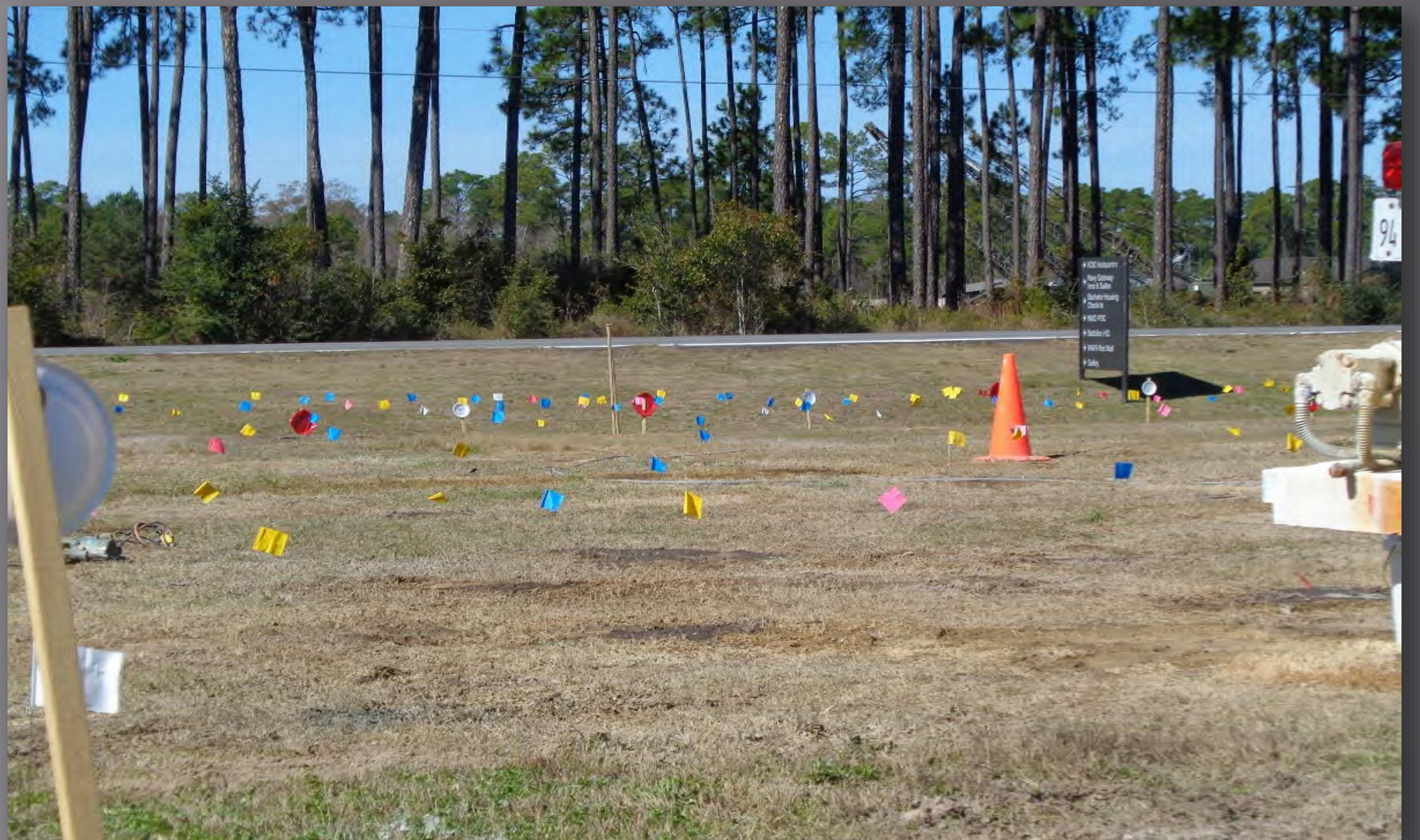
Injection Locations: Multi-colored flags show some of the 341 locations selected for BIOX™ injections at Site 6.
