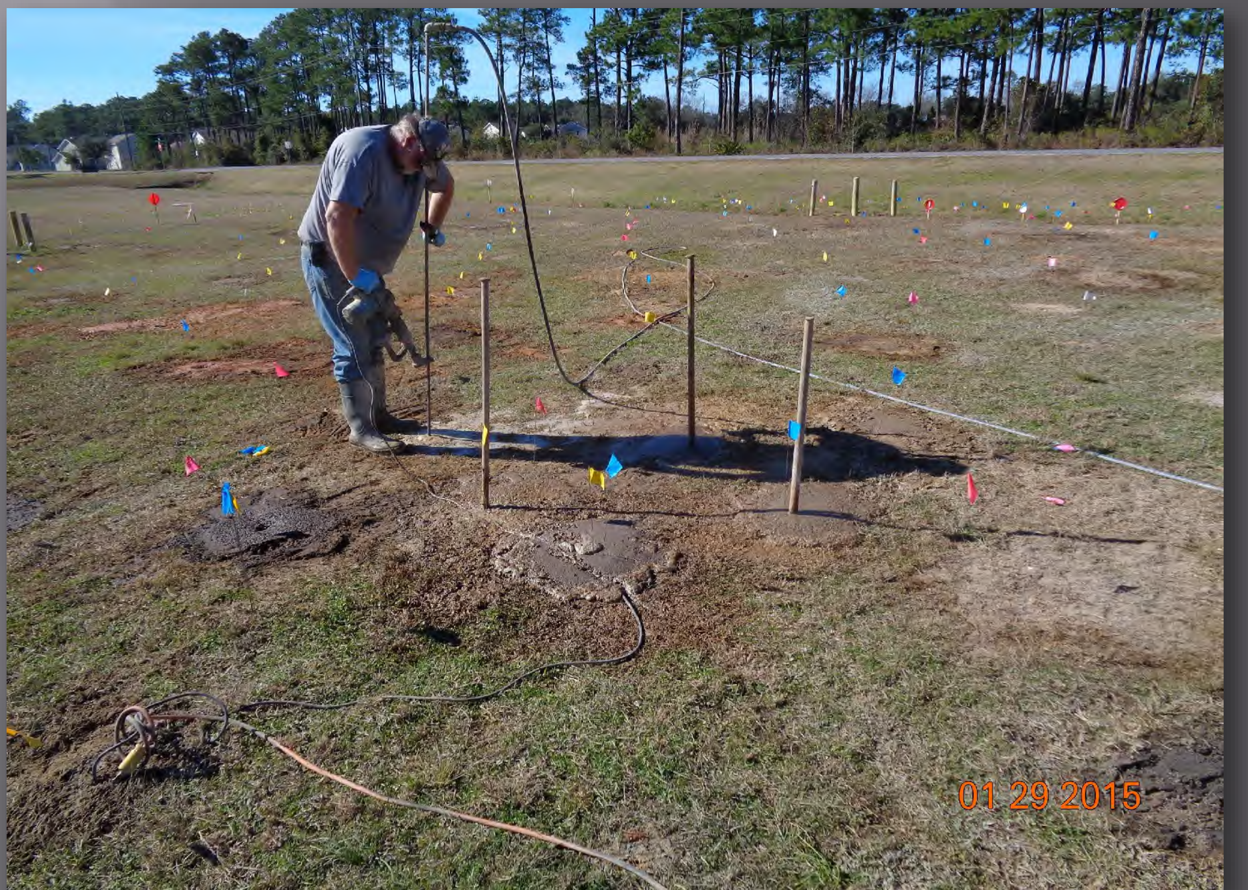
Injection Process: Over 10,000 pounds of BIOX™ were injected to depths of 2 to 9 feet in the contaminated area of Site 6.
