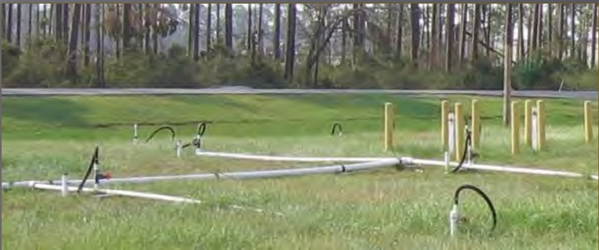
Surface view of the Multi-Phase Extraction System.
