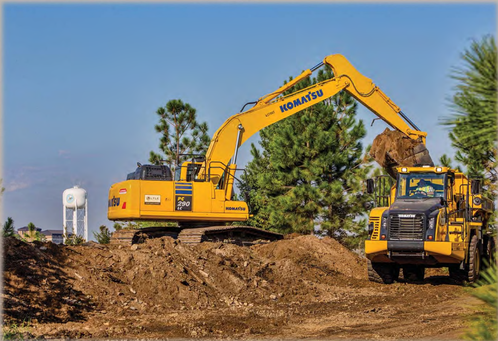
Stockpiled Sediment Loaded for Screening
