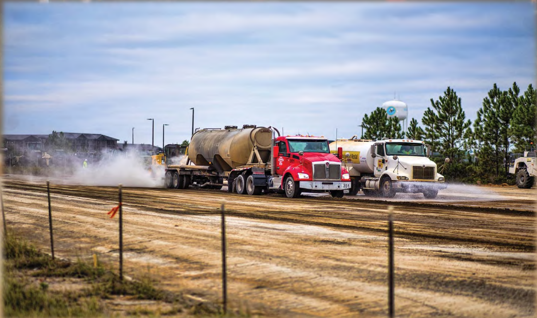
Applying Portland Cement to Sediment and Hydrating
