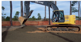
Contaminated soil was removed at Site 1.
