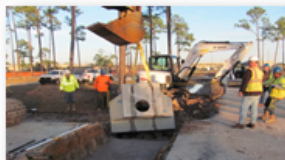
Construction of the headwall for a new culvert at Site 1.
