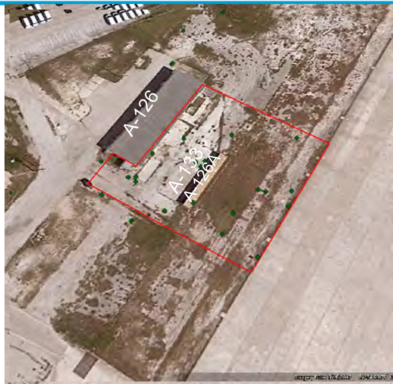
Wells remaining after abandonment
