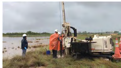
New Well (TFS-MW-18) Installation
