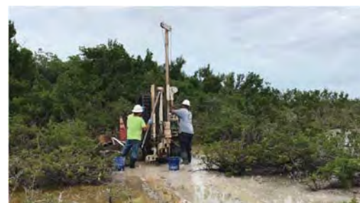
Piezometer Installation
