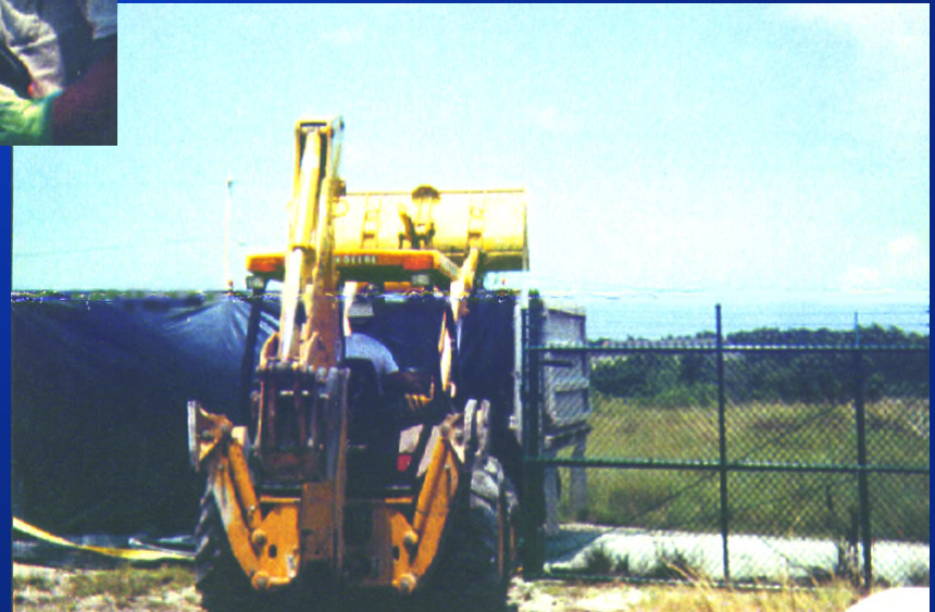
Loading of the PCB-contaminated soils for disposal
