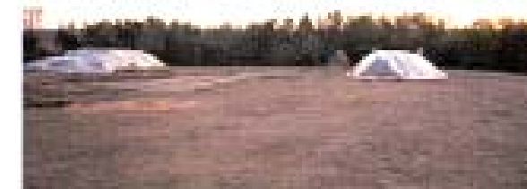
Area 31C – During Soil Removal
