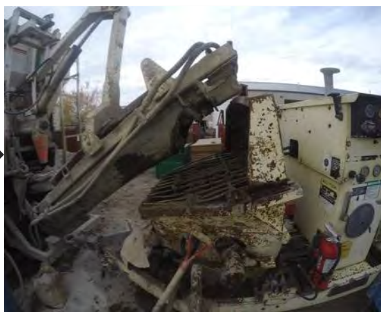
Deliver amendment into hopper and displacement pump
