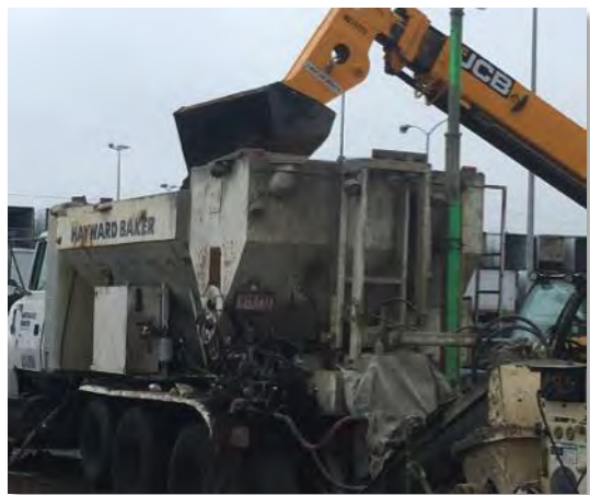
Batch-mix amendment ingredients in Elkin Mixer
