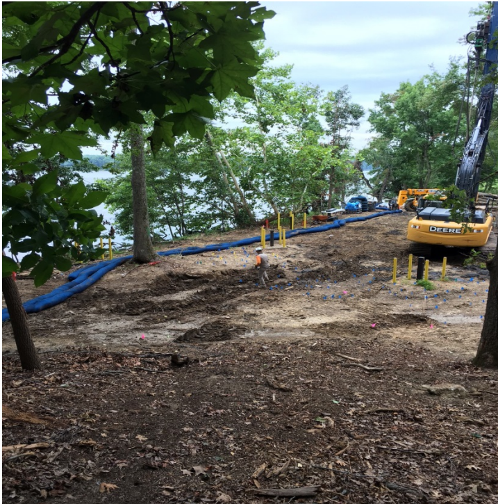
Erosion control tubing was placed along the edge of the site to prevent runoff during rain events.
