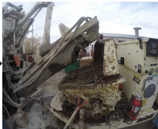
Deliver amendment into hopper and displacement pump
