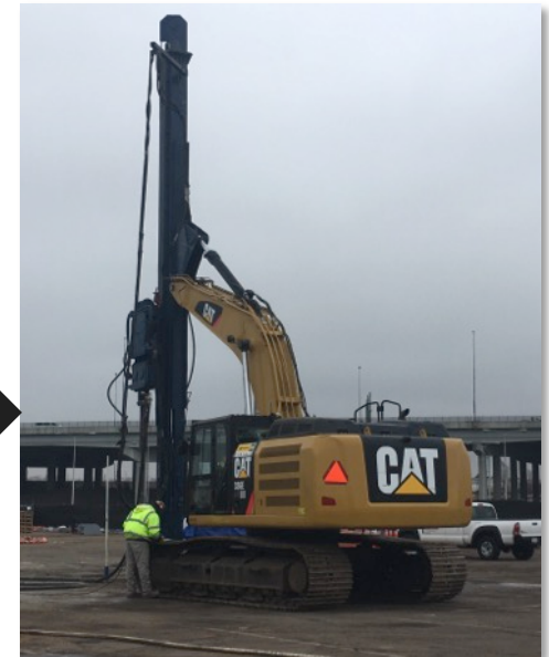
Pump amendment up mast and into mandrel for injection
