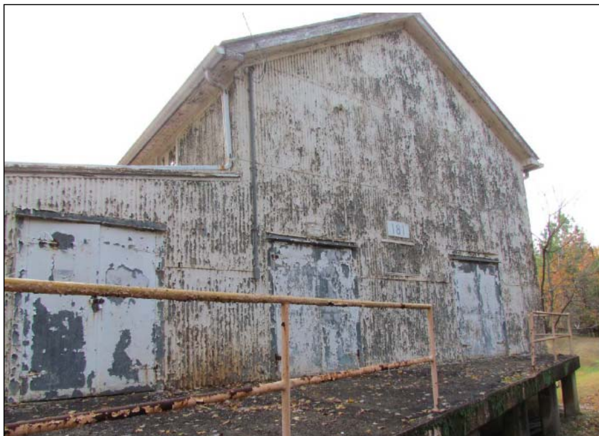
Photo of Building 181 on site with extensive paint deterioration on exterior walls and railings.
