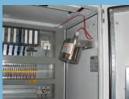
Self-Contained Aerosol Generators Testing
