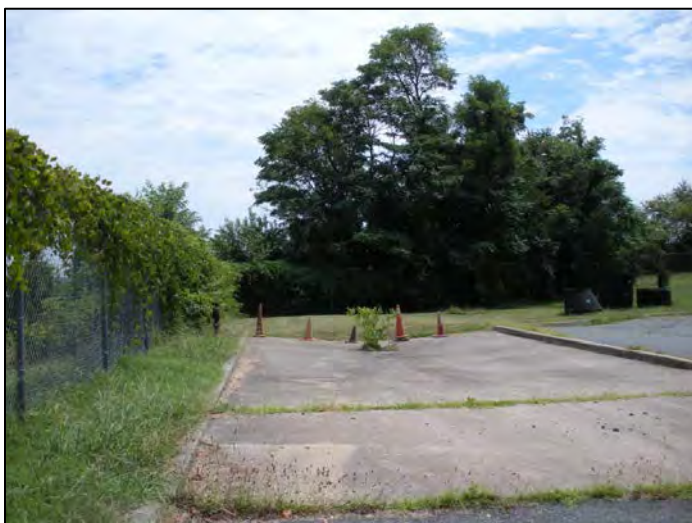
Figure 6: Site 104, Concrete pad (underground tank loading/unloading area), looking east
