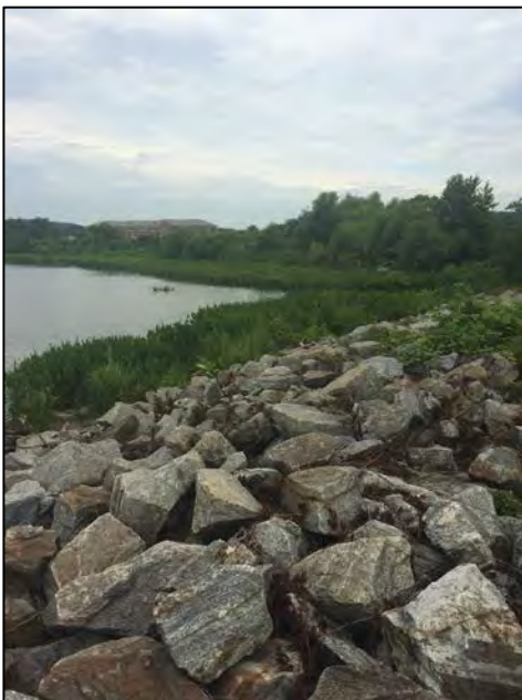
Figure 2: Site 4, Riprap along the shoreline with outlet of the constructed wetland in the background.
