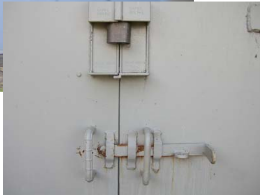
Existing 833 Padlock and NAPEC 0957 Hasp
