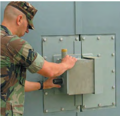
Universal mount ILD on double-sliding door
