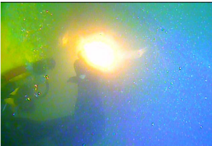
Figure 2: Diver cuts out deteriorated mooring chain.
