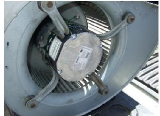
New ECM Green Motor Installed in Blower Prior to Demonstration
